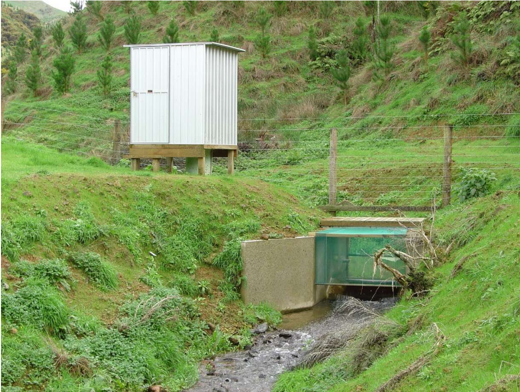
Figure 2. PW2 Weir and shed in July 2003
